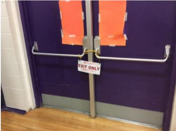
LH1 - Doors are currently being secured with a bungee cord. We recommend that the bar locking mechanism is repaired or replaced so that the doors are secured at all times.
