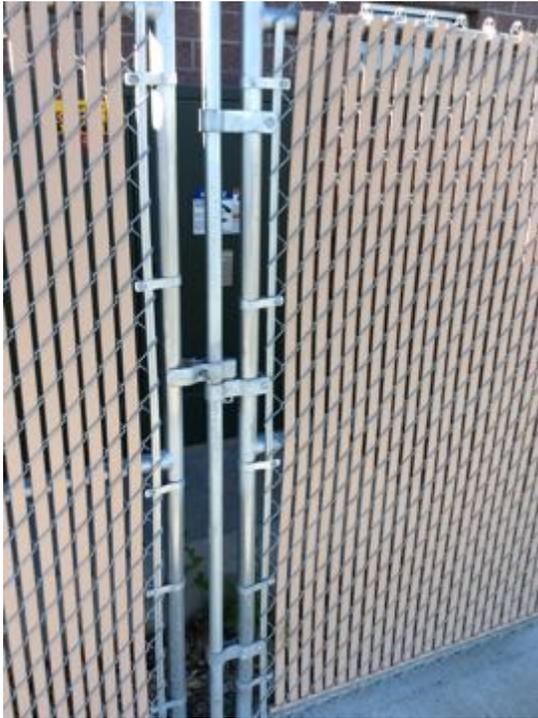
ST12 - Unsecured access to electric panel. A gate lock is needed like what is displayed in the next picture ST13.
