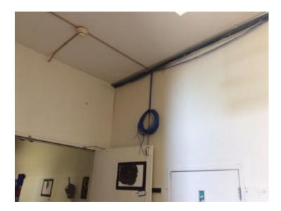
LH5 - Excess wire should be removed or enclosed in conduit to prevent access.
