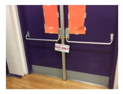
LH1 - Doors are currently being secured with a bungee cord. We recommend that the bar locking mechanism is repaired or replaced so that the doors are secured at all times.
