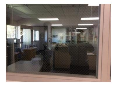
SD1 - Wire mesh windows provide an additional layer of security by forming another barrier that an intruder must overcome in order to gain entry into the room. We found wire mesh windows throughout the school district office.
