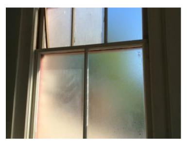
LH6 - Windows are currently held closed by a piece of wood that is positioned at the top of window. We recommend replacing these windows with either wire frame glass or the double pane windows found in many of the district's schools.
