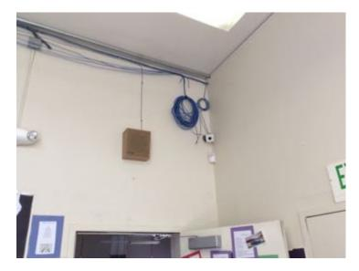
LH4 - Wires leading to the security camera should be enclosed in conduit to prevent access.
