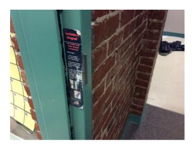
GP5 - Lockdown magnets were in place, covering the strike plate of most classroom doors. The magnets show signs of wear and may be in need of replacement.
