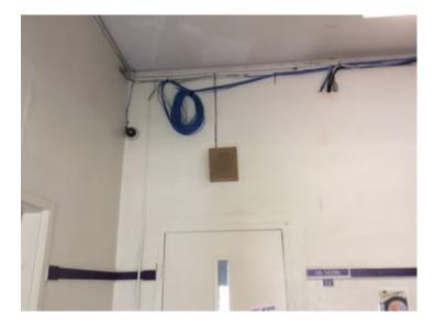
LH2 - Wires leading to the security camera should be enclosed in conduit to prevent access.
