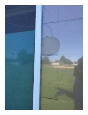
PP8 - Broken window on back of portable. This window should be replaced. Portable windows as well as all exterior windows on regular classrooms should have shatterproof window tinting.
